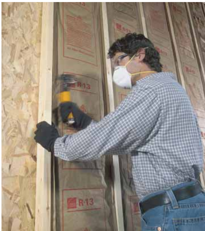
Owens Corning 3-1/2" Thick x 15" Wide Faced R-13 Insulation •40 sq. ft. roll •Ideal for insulating exterior walls, or any small project around the house •Helps control noise #13235
