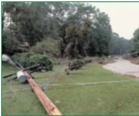
Stay away from downed or dangling lines, especially when clearing fallen trees.
