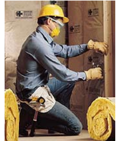
Adding insulation is a simple task that saves energy.
