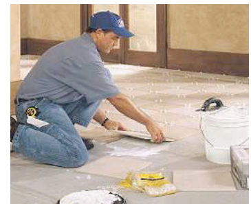
Find the center of two opposite walls and lay tile along the chalk lines.
