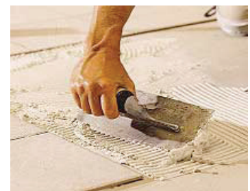
Spread the adhesive with the trowel's notched edge.
